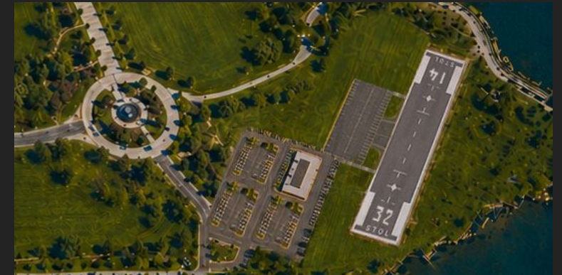
Closed municipal airports under redevelopment, such as Bader Field, Atlantic City
